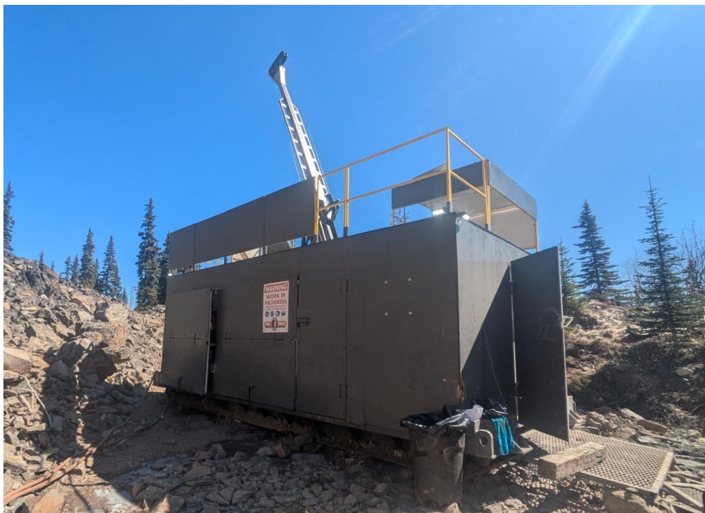
Image 1: Second drill rig on site at Getty North
